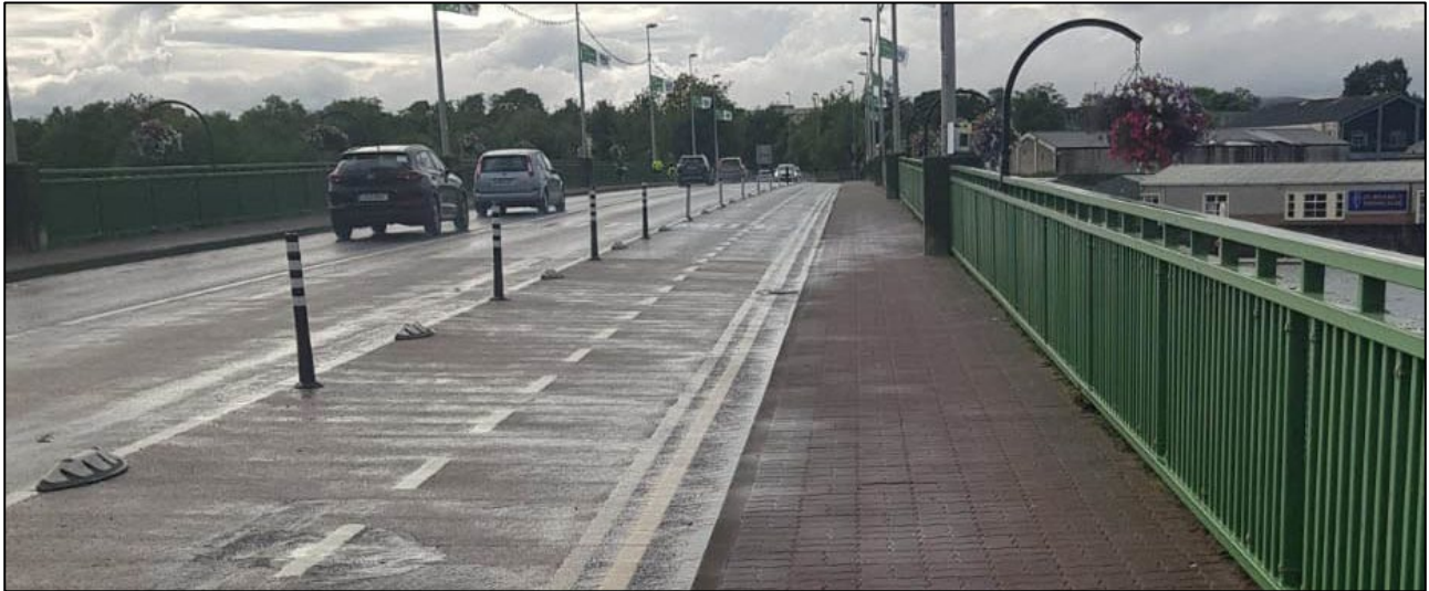
Figure 3-10 Shannon Bridge dedicated two-way cycle lane
